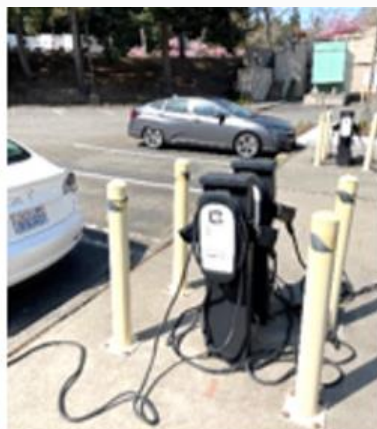
L2 EVSE located side by side to cut costs and power EVs on both sides.
