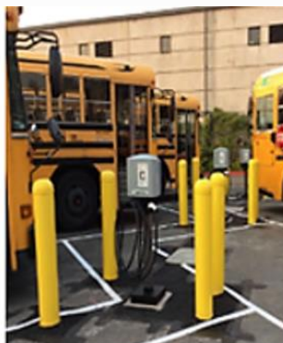
Single dual-port charging unit positioned to serve multiple vehicle parking spots. (Photo: Dept. of Ecology)
